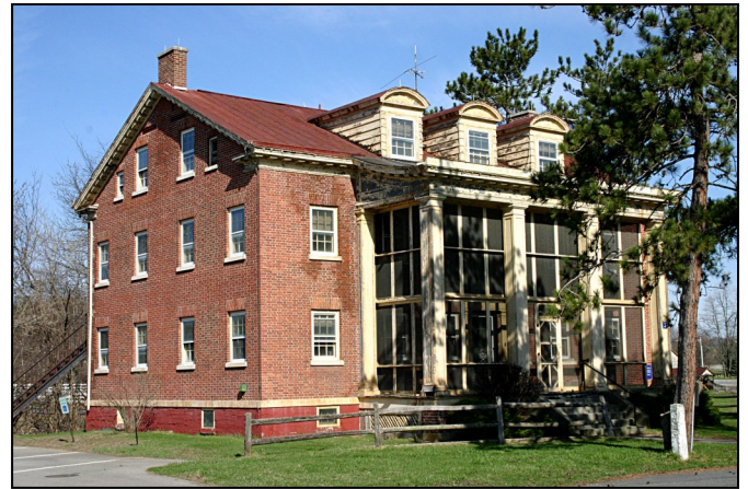
Colonial Revival style dormer windows and other details were added to the Brethren's Workshop and Trustees Office along with enclosed sleeping porches as part of the new development in the late 1920s.
